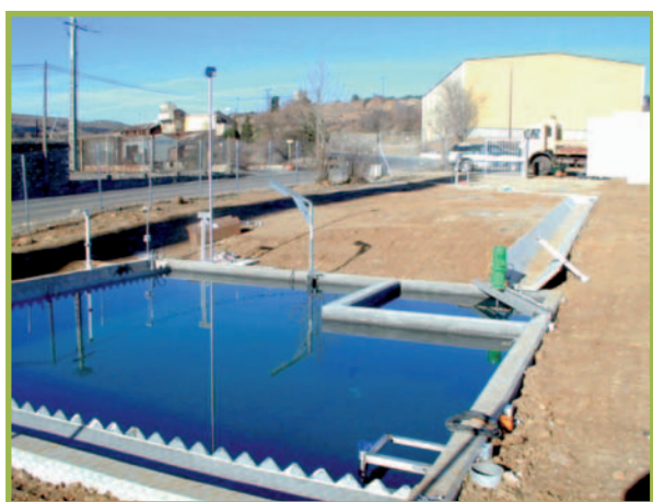
Figure 24 : on-line coagulation and flocculation.
