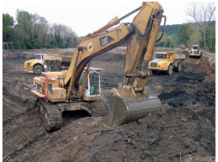
Figure 13 : Excavation of contaminated soil.
