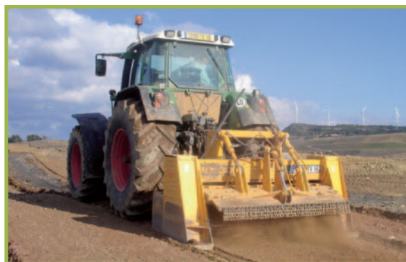
Figure 17: Mixing of steel shot with the soil.
